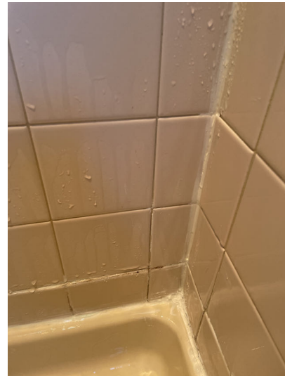
Damaged grout
