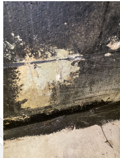
Efflorescence
