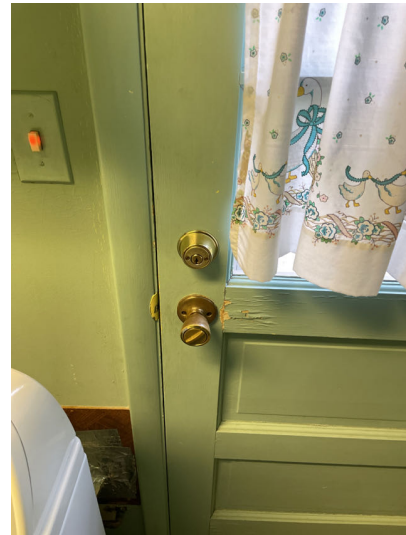
Laundry room: Interior keyed deadbolt
