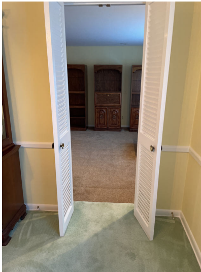
Dining room: dragging the floor
