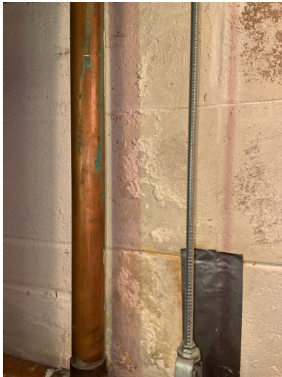
Efflorescence
