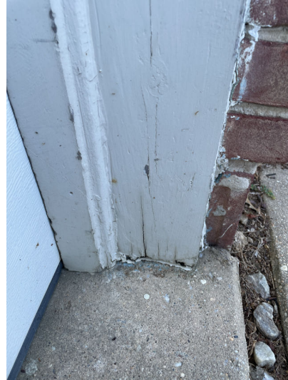
Wood deterioration
