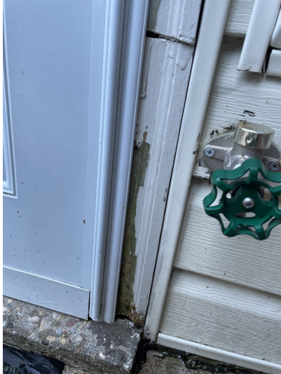
Wood deterioration
