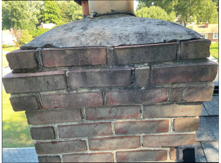
Mortar deterioration
