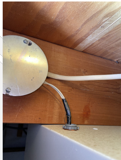
Improper wiring
