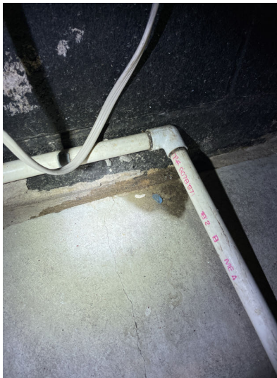
Condensation leak
